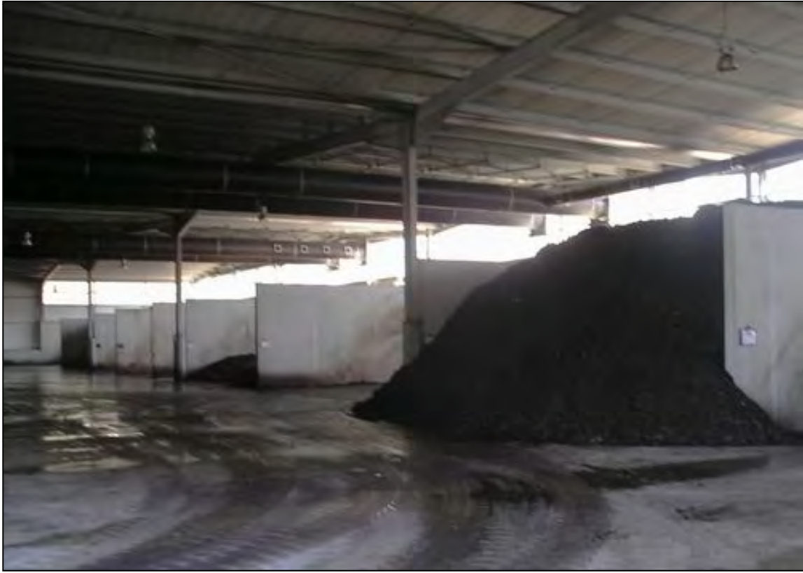
Photos 25 & 26 - Curing Bunkers in Shed
