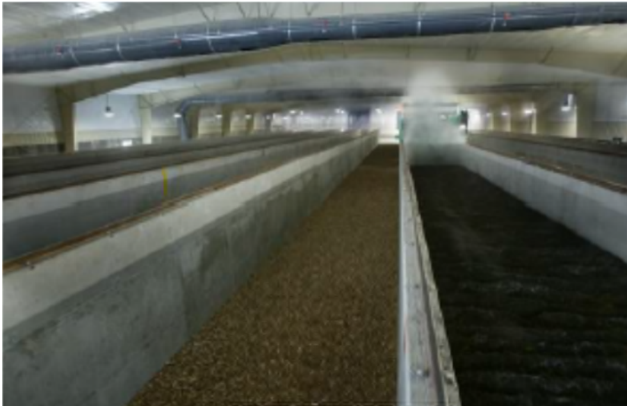
Bay Aeration system. Photo provided by BDP Industries.
