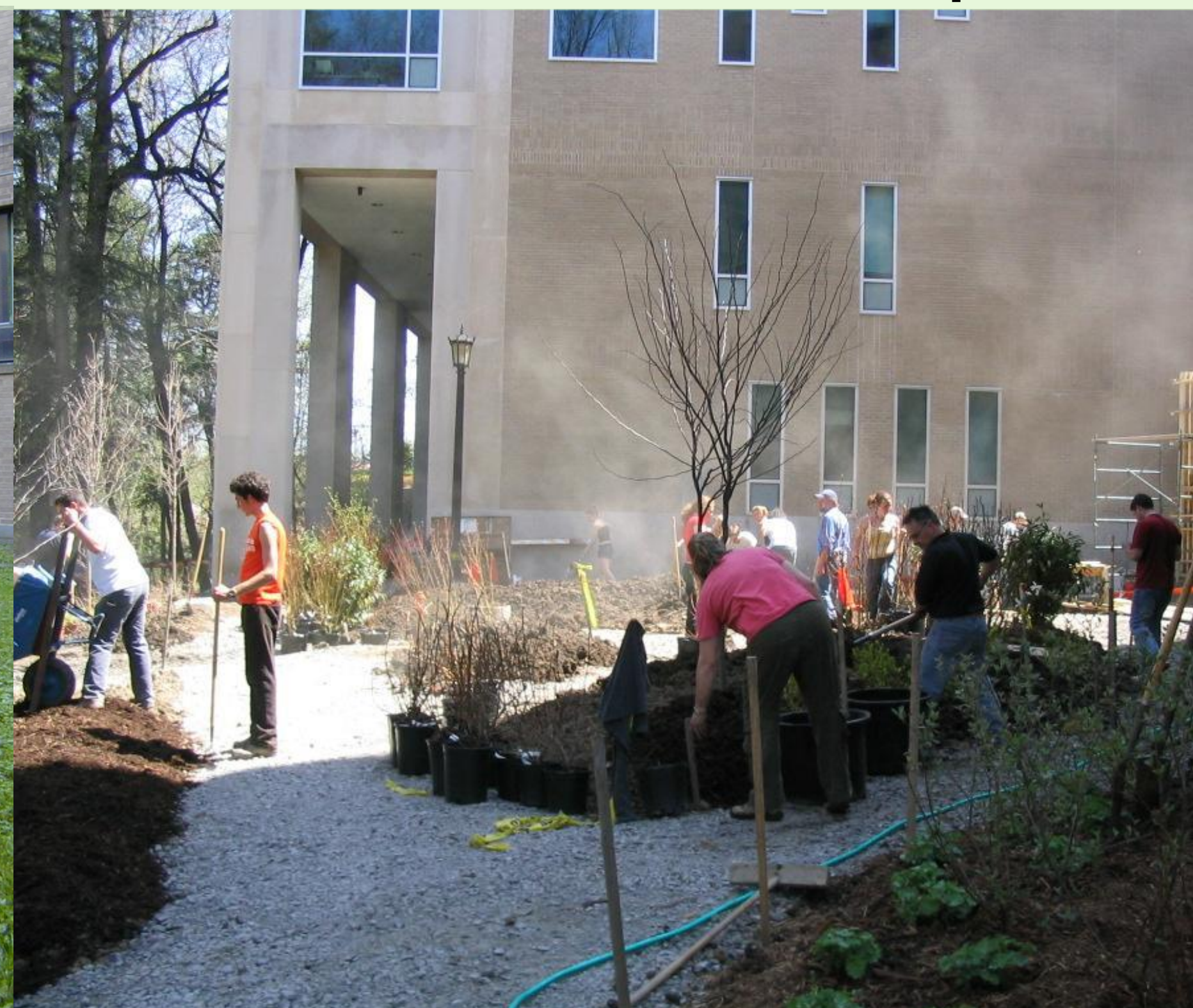
Construction-damaged soil removed and blended with compost to allow for healthy plant growth
