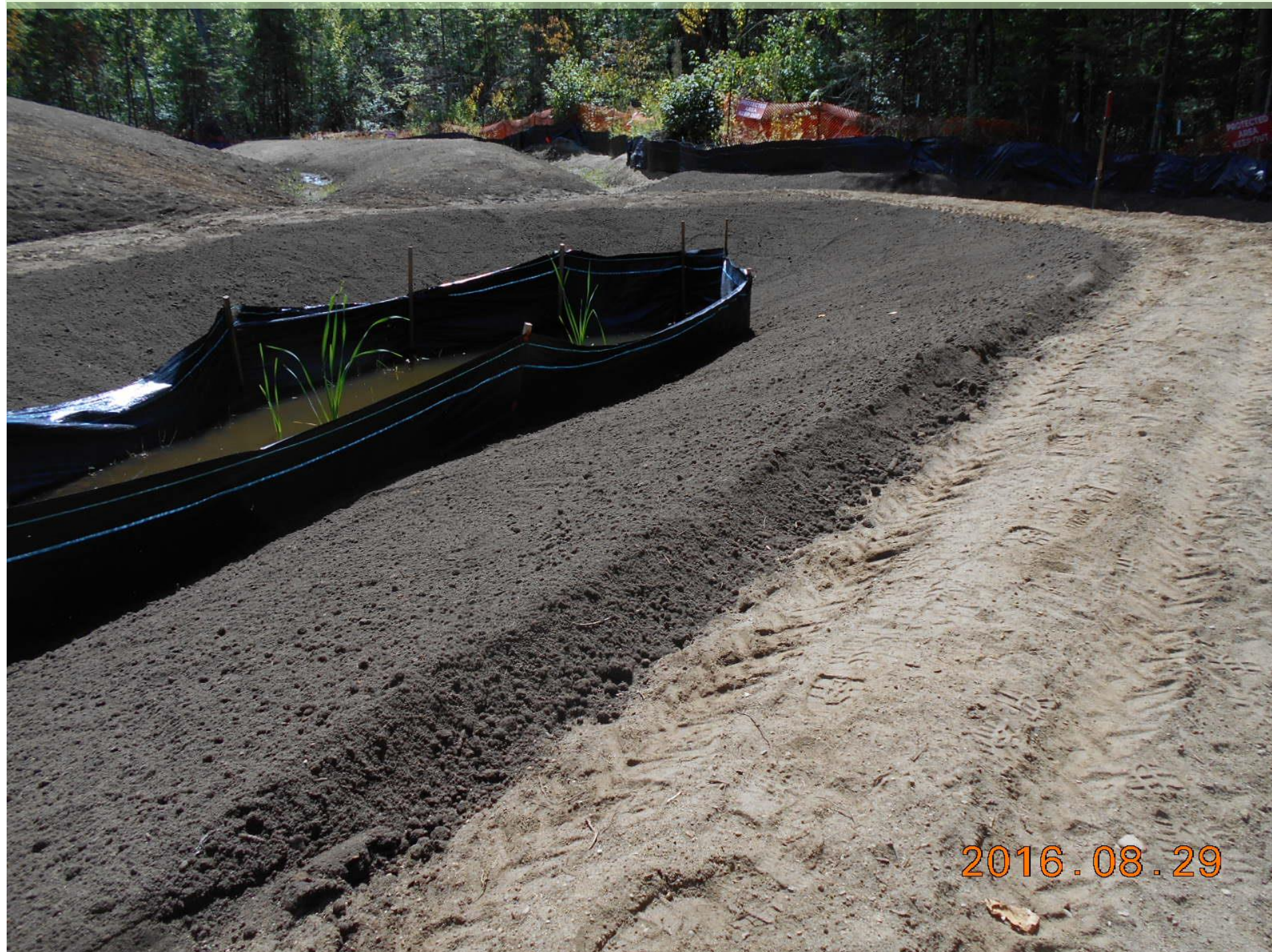
Blended soil placed and mulched with straw in September
